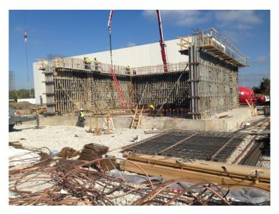
Trice completed construction of a new three bay transformer oil containment structure consisting of a 1400 cubic yard 2.5 foot thick mat slab and 30 foot high fire walls at the site of a new construction 345kv substation.
